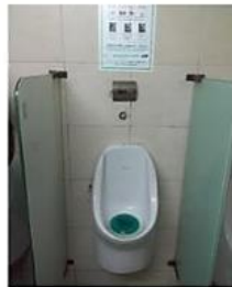
T.S. Pollution Control Board
