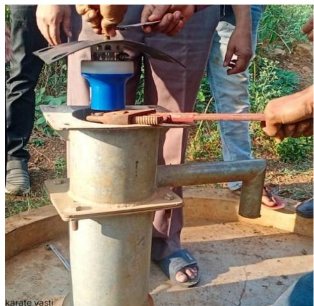
Installation of Taraltec reactor
