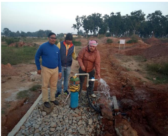
Installation of Bhungru which augments the groundwater
