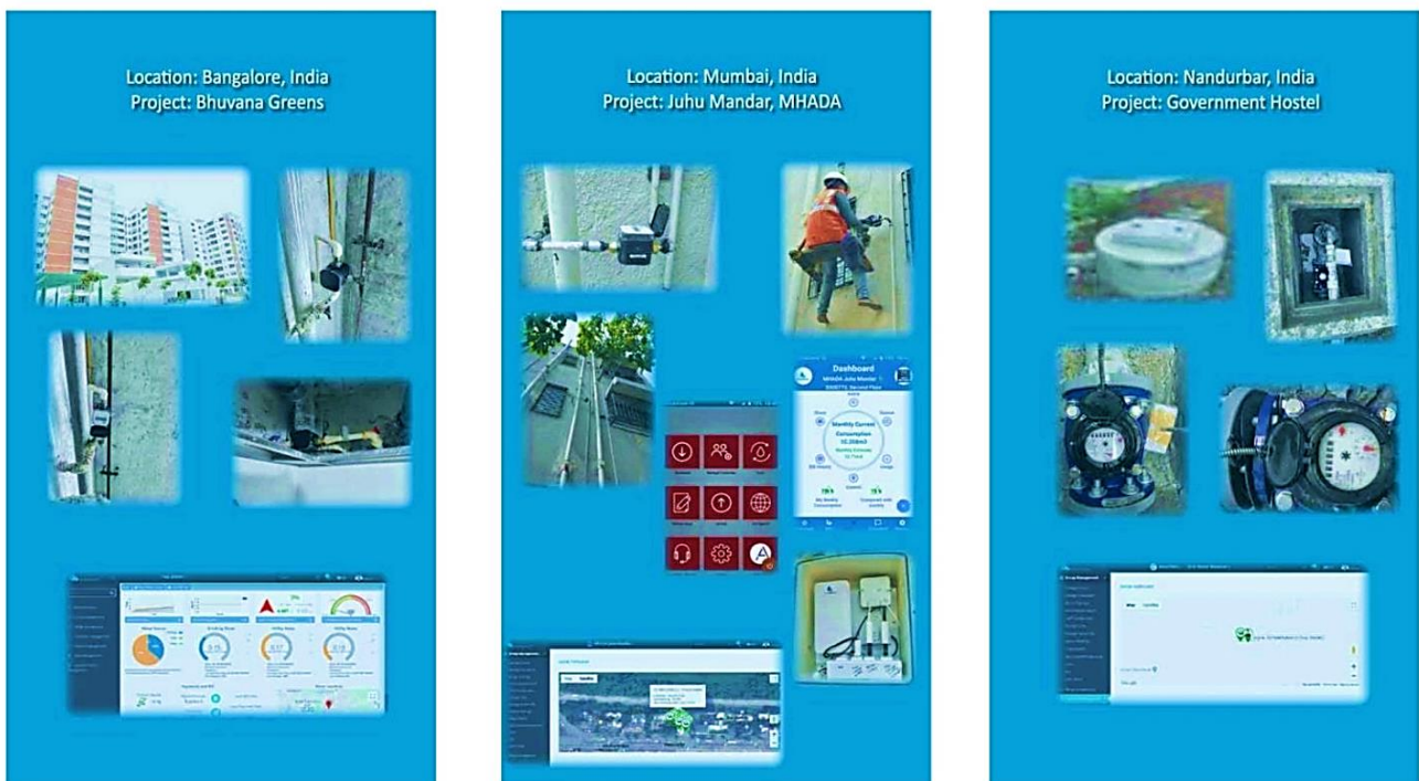
Installation of DBD water systems at various places
