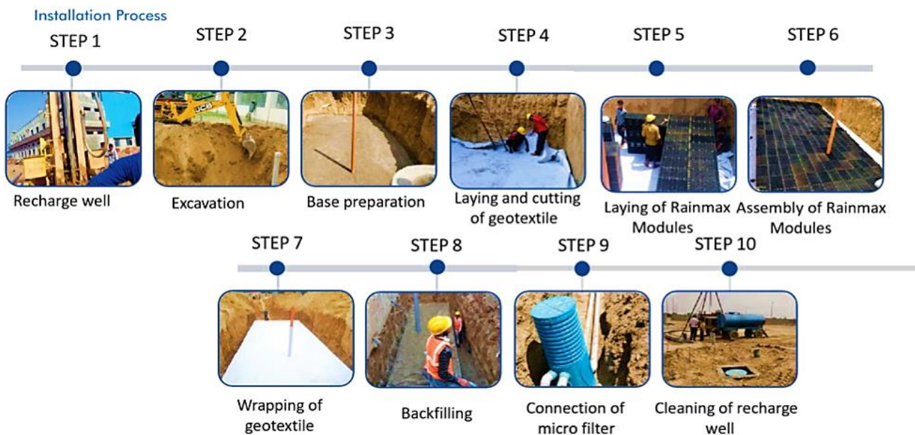
Installation Process of Rainmaxx modules on site
