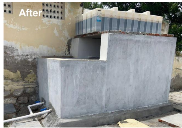
3KLD pilot plant for a community toilet containment in Trichy, Tamil Nadu.
